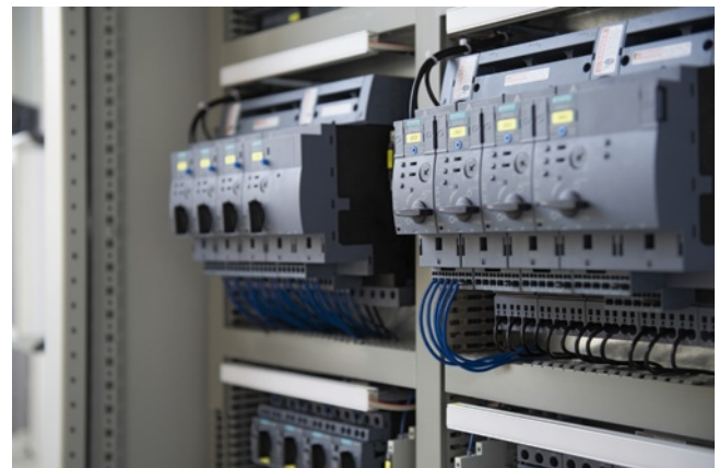
Connection of a motor starter group made up of three 3RA64 direct-on-line starters and a 3RA65 reversing starter
